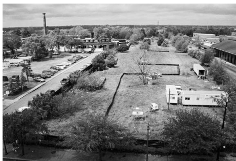
Crews remove lead and arsenic contamination from the recently acquired 9.5 acres.
