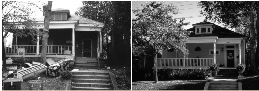
Most of Tatnall Square Heights' homes have been restored, including the one above, pictured before (left) and after (right).
