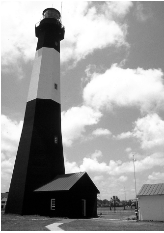
Tybee Island Lighthouse received a new coat of paint courtesy of Hampton Inn's Save-a-Landmark Campaign.
