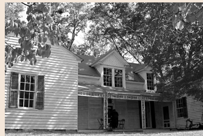
ROSSITER-LITTLE HOUSE , Sparta, c. 1800. One of the oldest homes in Sparta, the house was built by Dr. Timothy Rossiter. Contains many original features, including doors, mantels and hand-planed board walls and ceilings. Two front wings were added before the Civil War. NEW PRICE: $69,500. Contact Frank White at 404-885-7807.
