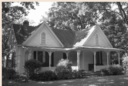
HOUSWORTH HOMEPLACE , Lithonia, c. 1890. 1,600-sq. ft. Folk Victorian home sits on nine acres near Arabia Mountain Nature Preserve. The 2BR/1.5BA house features four fireplaces, hardwood floors and original gingerbread detailing. Outbuildings include c. 1830 log kitchen, barn, log corner crib and a 1960s garage/workshop. Contact Frank White at 404-885-7807.
